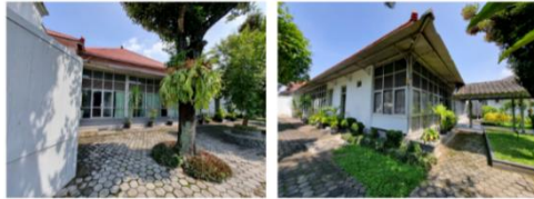
Figure 15. East and north existing facade Source: Author's documentation, 2025
